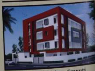
Lakshmi-Vishnu Smruti A 3-BHK Apartment Scheme in Progress at Khare Town, Dharampeth, Nagpur. Flats for Sale
